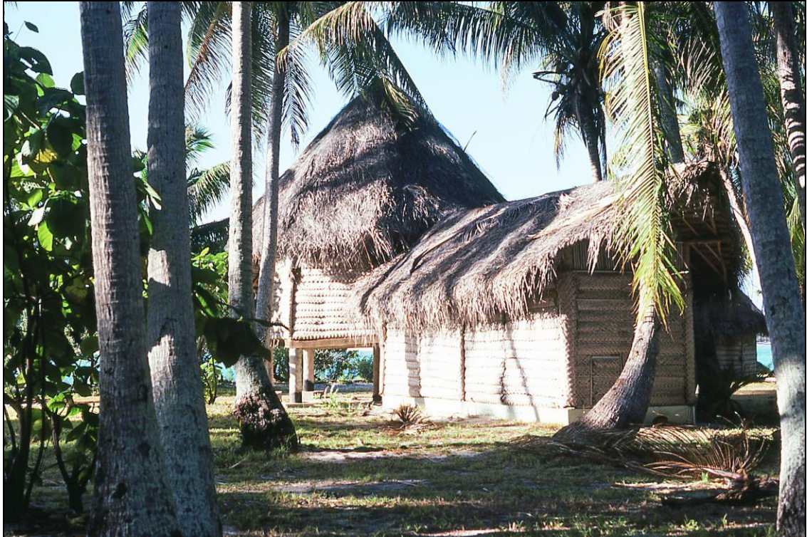
Exterior construction of fare; front section on stilts is bedroom, rear is bathroom
