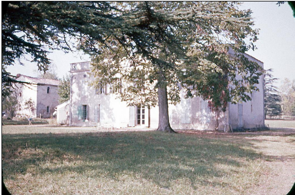
Rear view of Château de Labarthe, looking toward patio and French doors to dining room
